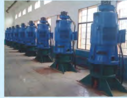
洞庭湖水利工程永丰泵站 Dongtin Lake Water Conservancy Project
