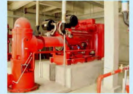
首都机场柴油机立式长轴消防泵组 Diesel Engine Vertical Turbine Fire Pump Set in Capital Airport
