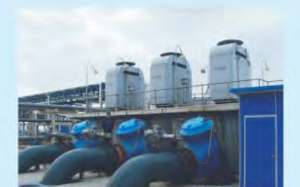
中海油和邦化学立式长轴海水泵 Vertical turbine seawater pump for CNOOC Hebang Chemistry
