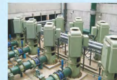
浦钢热轧ACC立式长轴泵 Hot rolling ACC vertical turbine pump for Pudong Steel
