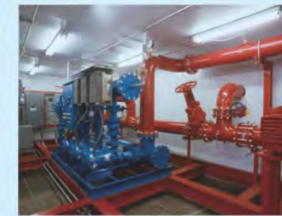
孟加拉AKG水处理站工程 AKG Water Treatment Station In Bangladesh
