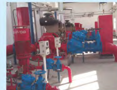
宁夏炼油柴油机消防泵 Sinopec Ningxia Refining Diesel Engine Fire Pump
