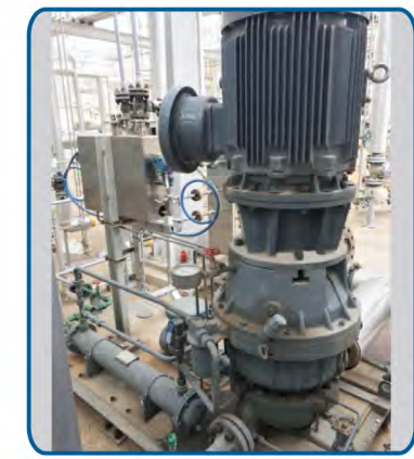
▲ SINOPEC YANSHAN PETROCHEMICAL CO.,LTD C4 Feed Pump Flow : 22m 3 /h Head: 646m Motor power: 75 kW
