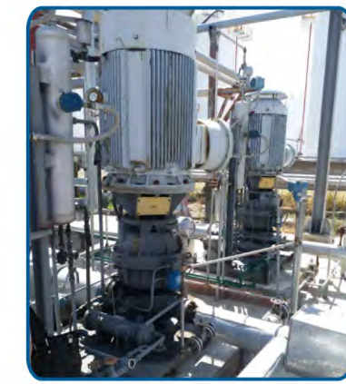
▲ CNPC DUSHANZI PETROCHEMICAL COMPANY Ethylene Feed Pump Flow : 51.5m 3 /h Head: 615m Motor power: 132 kW
