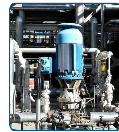
▲ SHANXI YANCHANG PETROLEU (GROUP) CORP. LTD Water Injection Pump Flow : 12m 3 /h Head: 820m Motor power: 110kW
