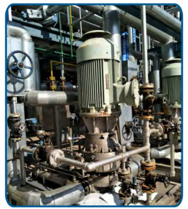
▲ CNPC WULUMUQI PETROCHEMICAL COMPANY Low Pressure Feed Pump Flow : 32m 3 /h Head: 300m Motor power: 55 kW
