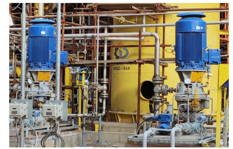
▲ CNPC DUSHANZI PETROCHEMICAL COMPANY Ethylene Feed Pump Flow : 51.5m 3 /h Head: 615m Motor power: 132 kW
