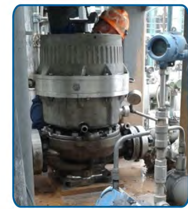
▲ CNPC LUOYANG REFINERY PTA Feed Pump Flow : 52m 3 /h Head: 1072m Motor power: 315kW
